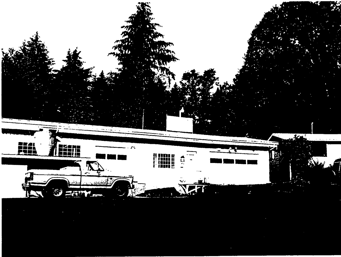
Composite of two photos below: "shop" to the left, "office" in the center and "garage/storage" to the right.
